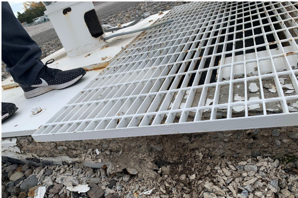
Photo 12: Significant concrete deterioration on Effluent Pump Station No.1 wet well.
