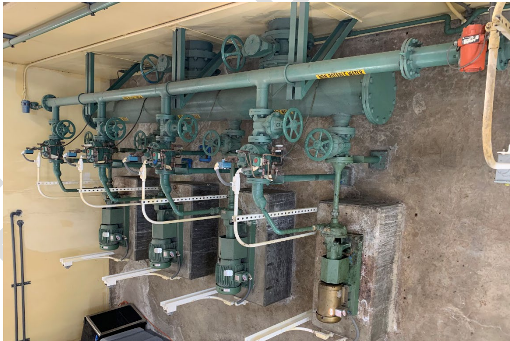
Photo 10: The 26-year old NPW pumps are fast approaching the end of their estimated useful life. The exposed pressurized header leaks periodically.
