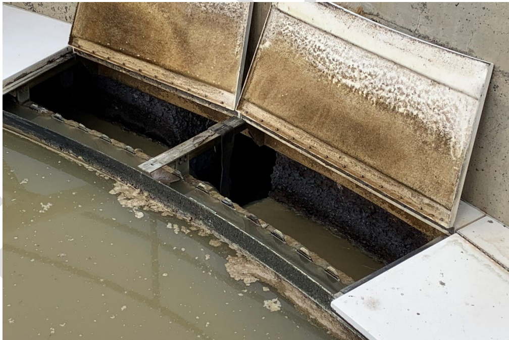
Photo 4: Significant mortar deterioration and exposed aggregate in the headspace of the concrete launder wall of Primary Clarifier #2.
