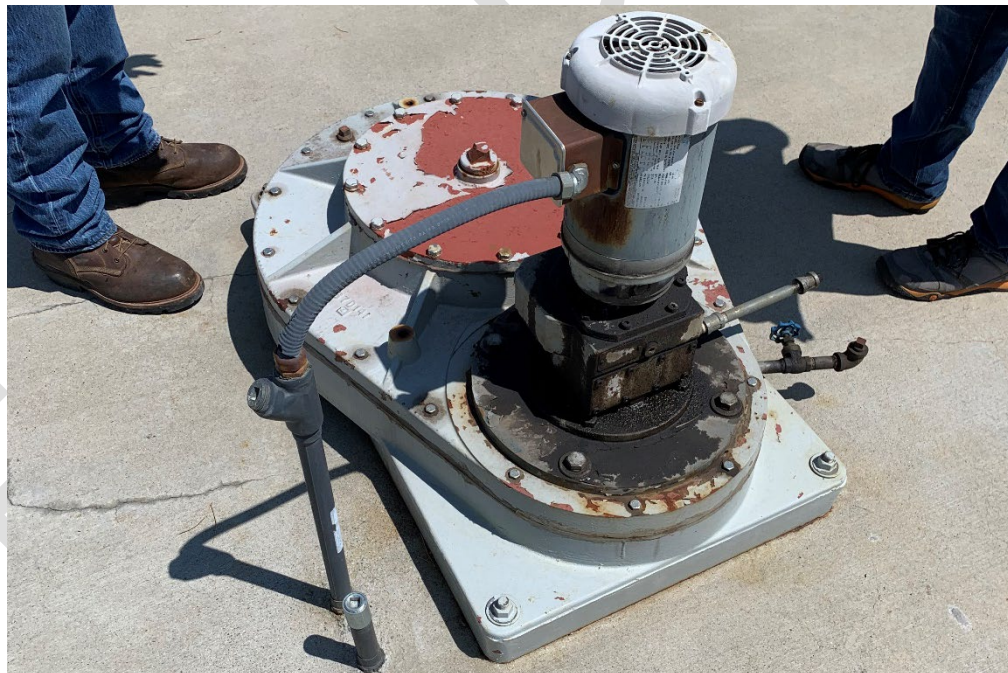
Photo 2: 20 year-old forced vortex grit removal unit drive pictured. It is currently offline due substantial deterioration from abrasive grit.
