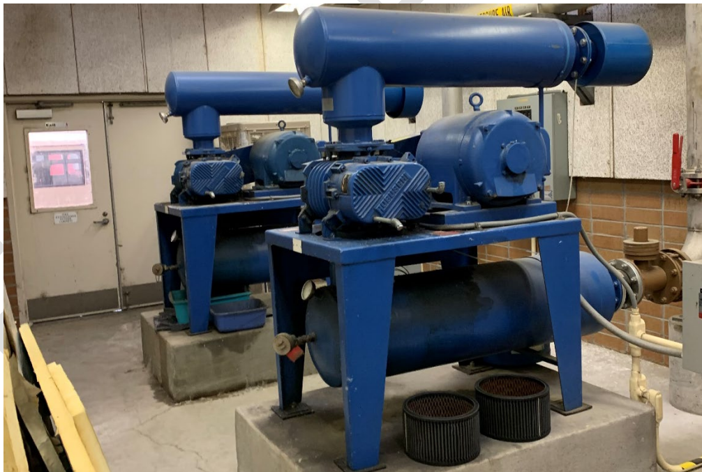
Photo 6: 25 HP positive displacement blowers, in the sludge thickening building, require periodic repairs, but are in good working condition.
