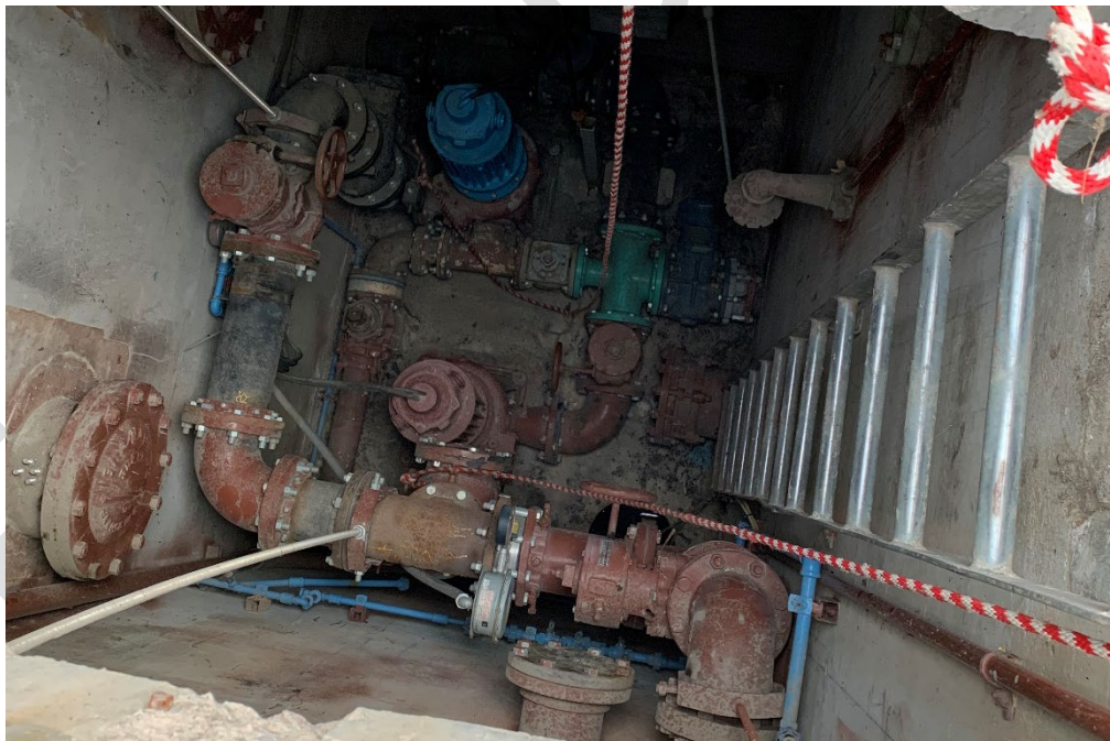
Photo 8: Existing gravity belt thickener feed pumps, approximately 30 years old, which operate in a one duty, one standby arrangement. Plant staff recently replaced the motor (blue colored) for one, while the other one requires a comprehensive rehabilitation or replacement.
