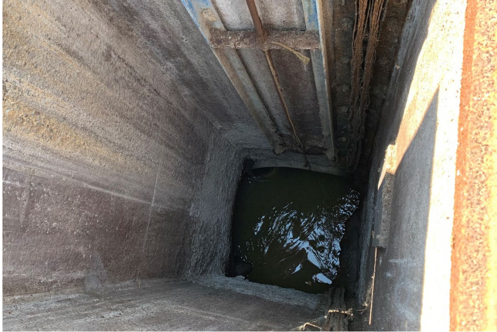
Photo 1: Influent sewer junction structure, upstream of the Headworks structure, with surface aggregate exposure and metallic corrosion.
