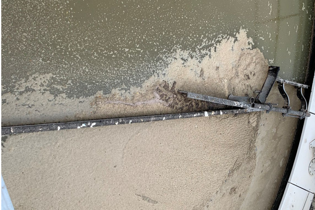
Photo 3: Significant visible corrosion on clarifier mechanism, skimmer arm, of Primary Clarifier #2.
