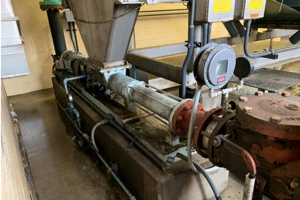
Photo 7: The 26 year old thickened sludge pump, located inside sludge thickening building, is past it's useful life and is no longer reliable. It requires frequent maintenance to maintain beneficial use.
