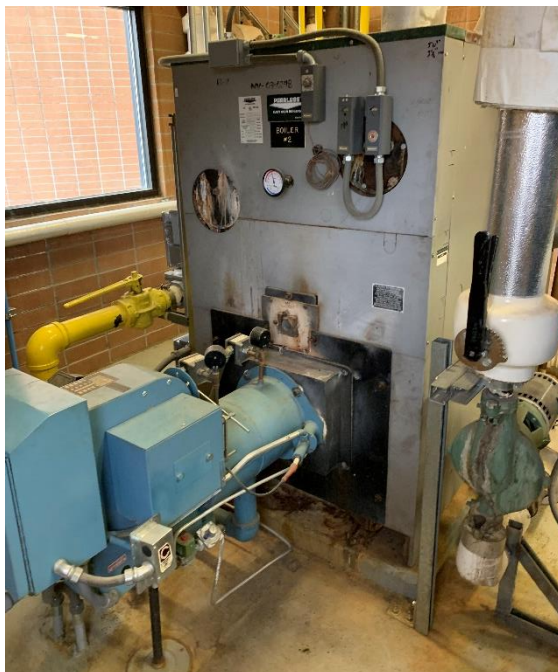
Photo 9: 25-year old Boiler #2 recently inspected by QCS, noticed pitting on the plates.
