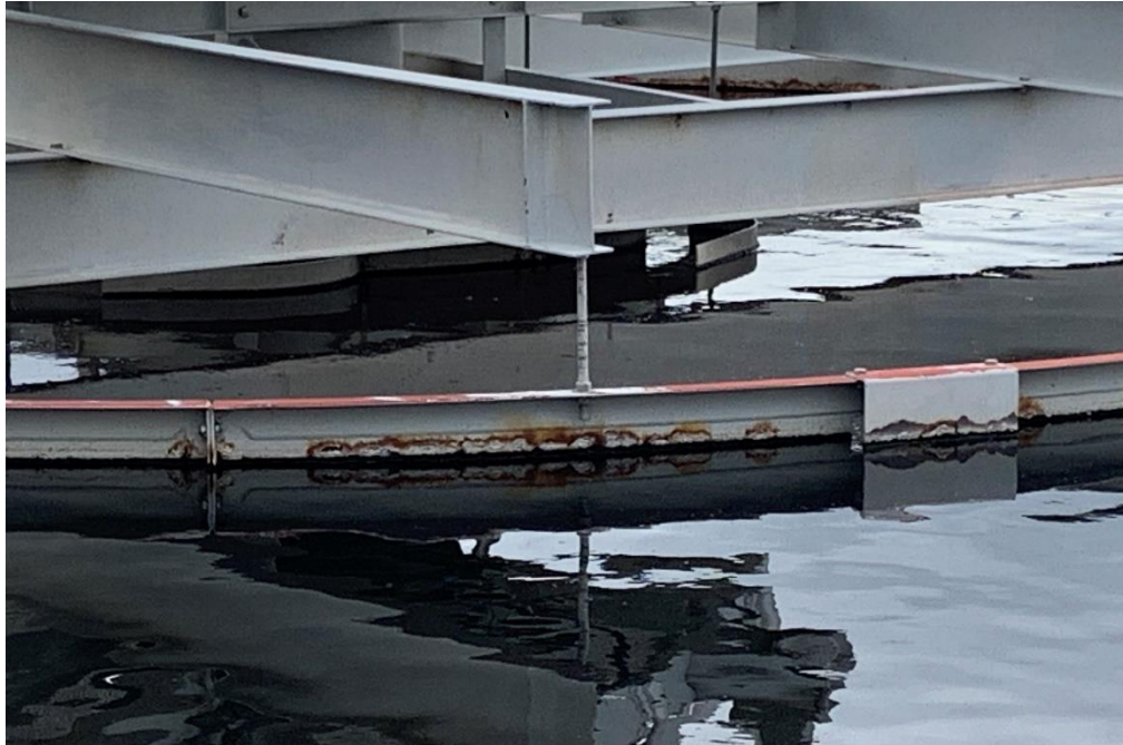
Photo 11: Operational secondary Clarifier #3, commissioned in 2000, displays corrosion and coating degradation.
